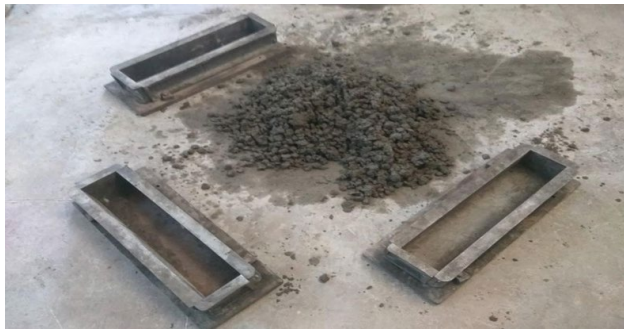
(a) Beam moulds prior to filling of concrete
